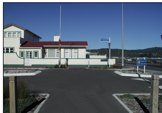
Figure 3. Pedestrian-vehicle space with tactile surfaces removed
